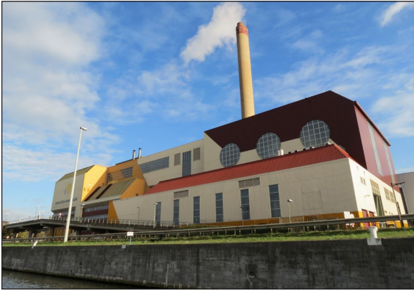
Verbrandingsoven in Neder-Over-Heembeek
